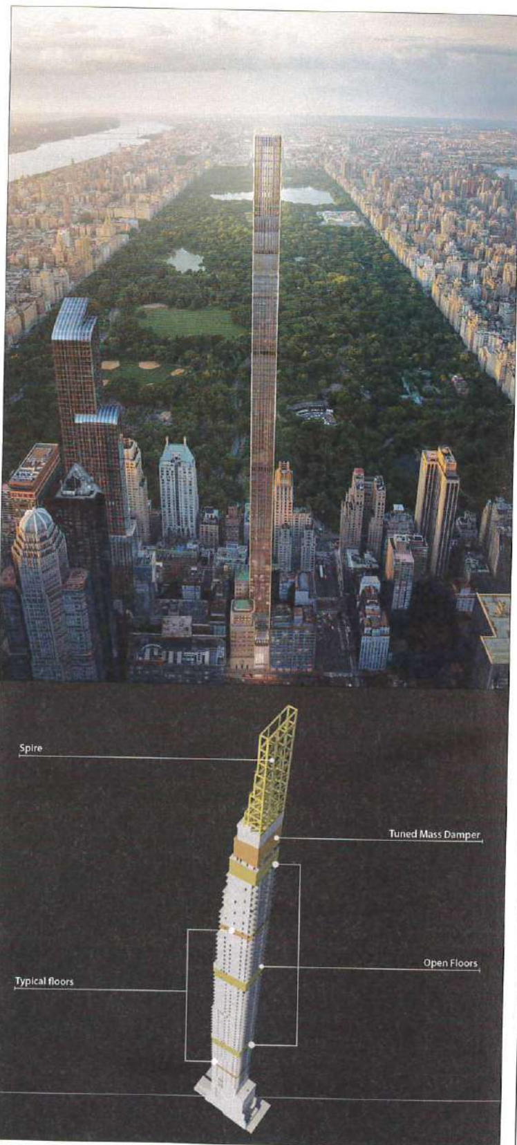
(Top): A rendering of 111 West 57 th Street. Its aspect ratio of 24:1 will make it the world's most slender building. (Bottom): Shear walls run the full length of the east and west exteriors and have been thickened to as much as one metre. Like 432 Park Avenue, it also has open floors that the wind will pass through to reduce vibration
